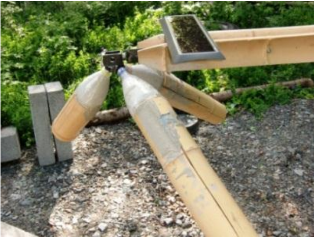
Space frame structure for solar panels
